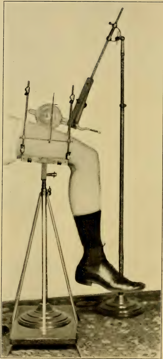
PLATE 62.—Author's Examining Frame and One-Minute Localizer, with middle of thigh in position for either simple examination or the simultaneous location of any lesion or foreign body. With the frame and part in this position sit in front of the frame, clamp the fluoroscope on the posts and inspect in the usual manner. Note that the frame holds the radial axis fixed and any part of the leg from the hip to the heel can be rapidly passed through the field of the non-distorted rays for successive examination. No other equally simple method exists.
